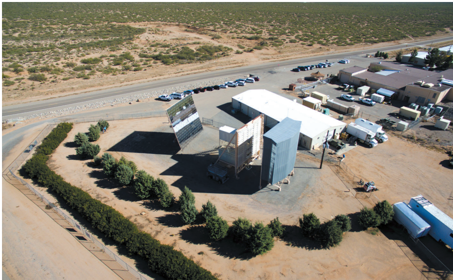
An aerial view of the solar furnace in operation. The heliostat can be seen directing sunlight through a shutter used to turn the furnace on and off.
