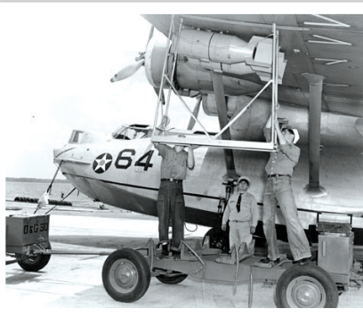
A seaman and a second class petty officer remove the bomb placement platform from the wing of a PBY Catalina aircraft under the watchful eye of a chief petty officer in 1942.
