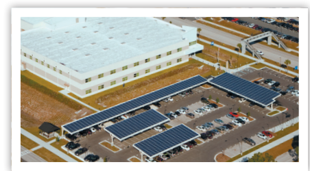
NAS Jacksonville energy conservation initiatives are found all over of the base. This photos shows flat-plate, solar-thermal collectors or “panels” on the roof of the parking lot of the P-8A ITC.
