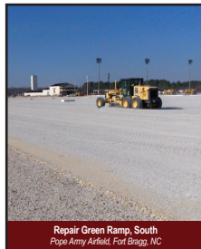
Repair Green Ramp, South Pope Army Airfield, Fort Bragg, NC
